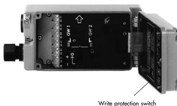
Fig. 3 · Type 3780 Positioner with opened cover
